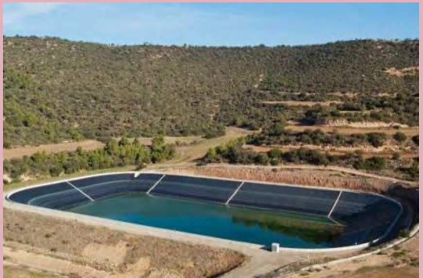
Irrigation pond of the Aigües Del Segarra Garrigues Irrigation Community.
